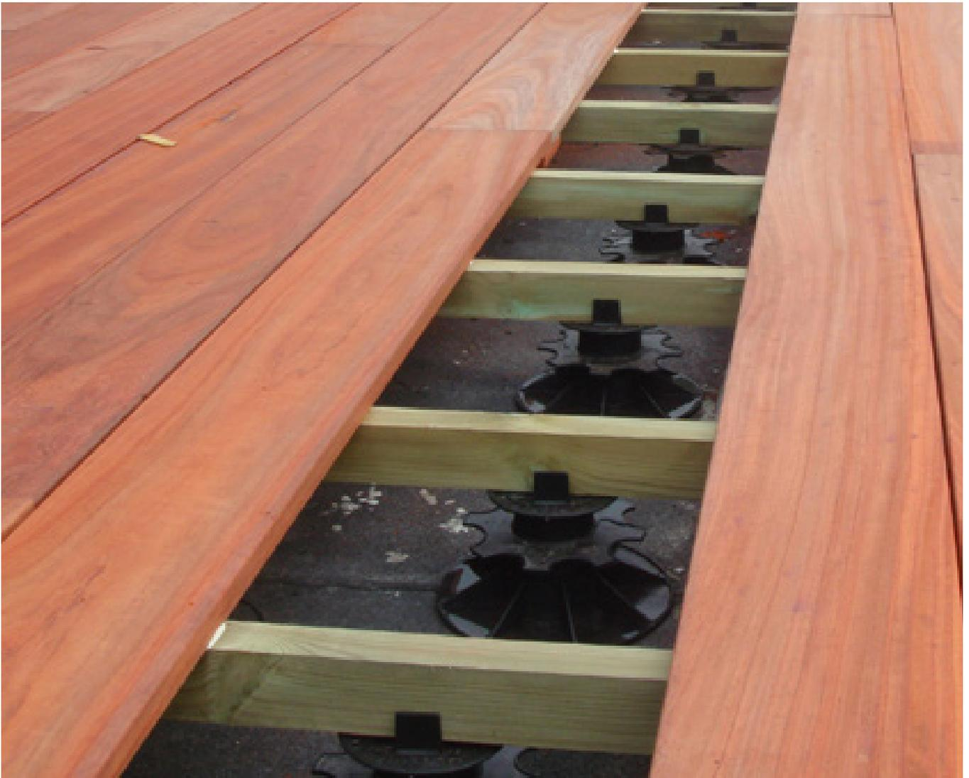
Use the recommended guide below to calculate how many Pavetuf Adjustable Risers you will need for your installation.
